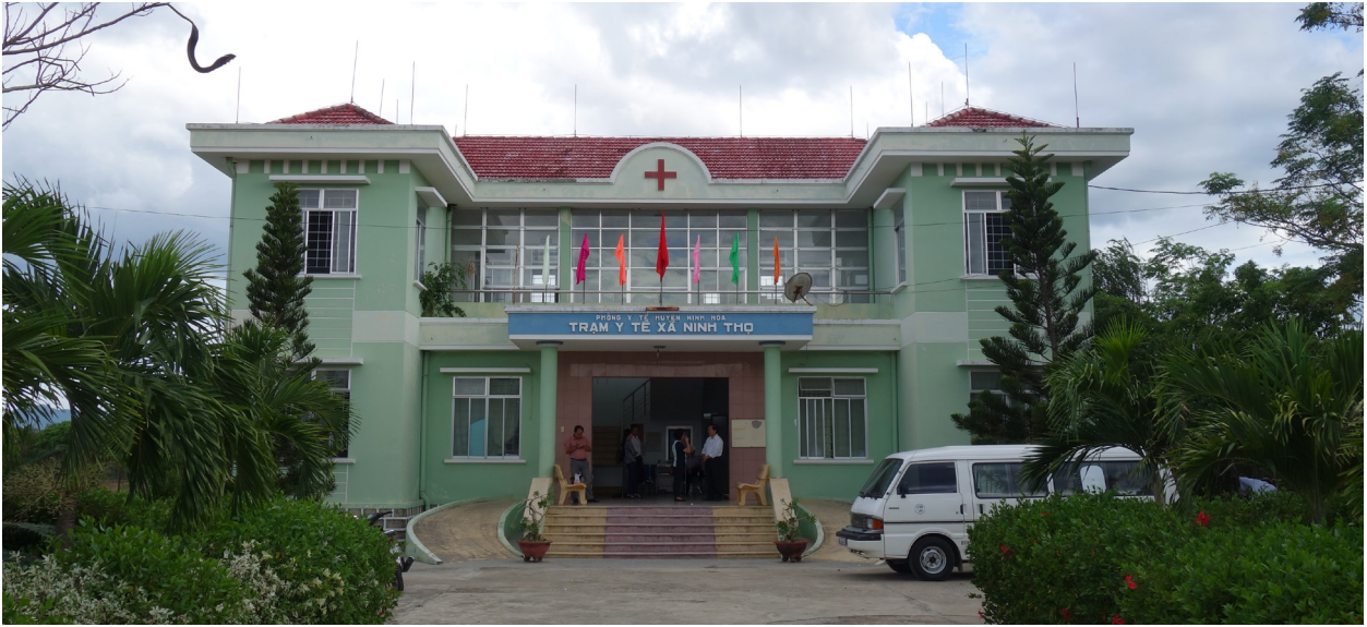
Above. A view of the front of a commune health center in Khanh Hoa. Pilot facilities generated community pride, and citizens actively participated in the construction process.
