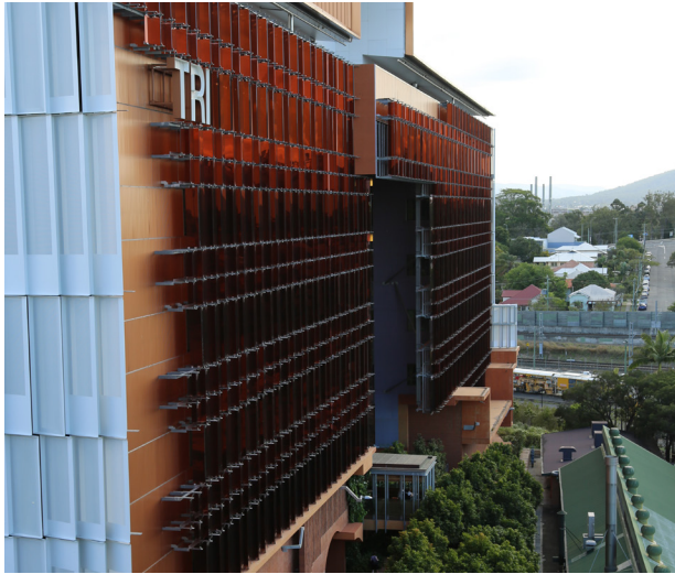
Above. The building's façade provides a much needed barrier to the intense heat and sun of Queensland.
