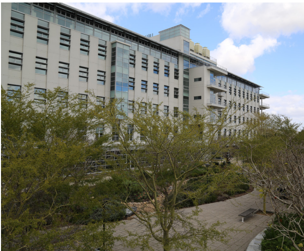
Above. The six-story laboratory building at the edge of campus overlooks part of the Cape Flats Nature Reserve and is easily viewed from a major Cape Town thoroughfare.
